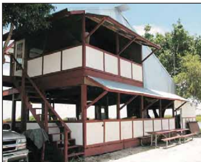
C. Open-Air Pavilion Mack's Fish Camp (DA1148)
