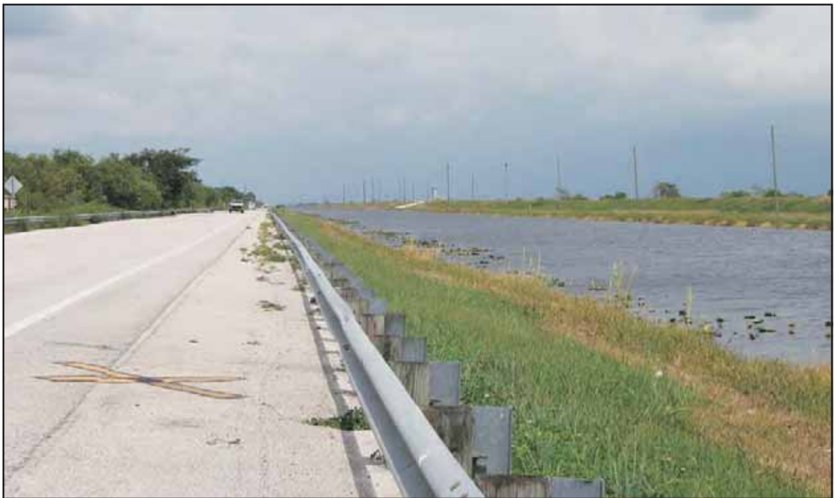
B. Tamiami Trail and Canal, Looking West
